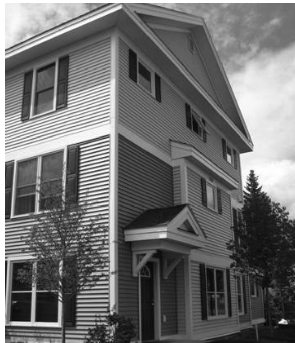
This transitional living facility in Manchester, NH is the nation's first multifamily residence to achieve a Platinum LEED certification.
